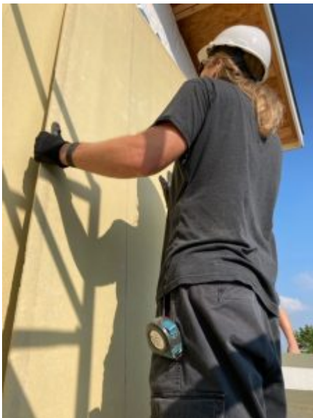
Hanging up siding at a HFH house in Austin
