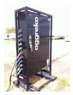
A Distro Panel with 3 Phase Tails connected to a generator — most connections use camlock
