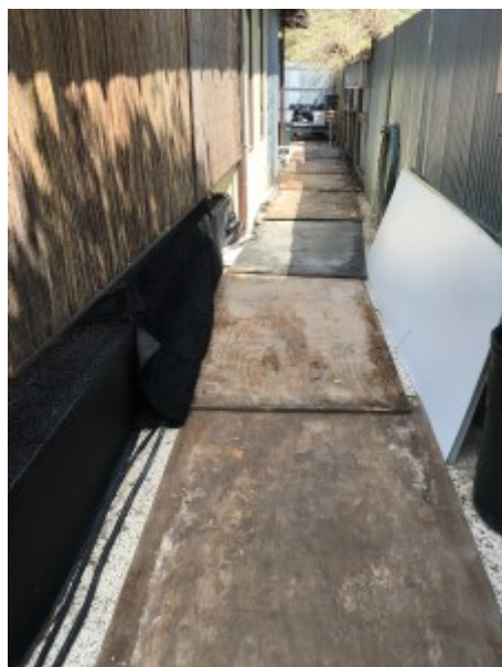
Notice how the plywood sheets overlap just a bit so it's easier for road cases to move along the path
