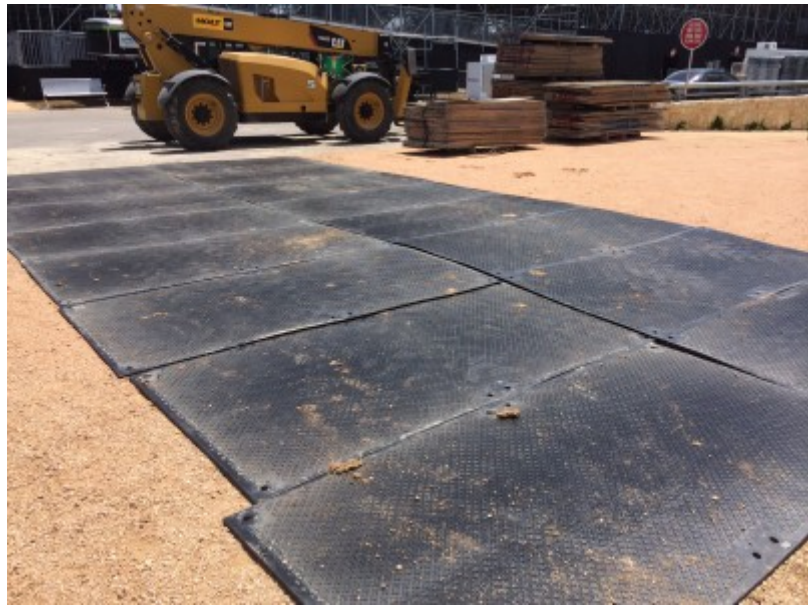
Reusable plastic 4 x 8 ground protection mats
