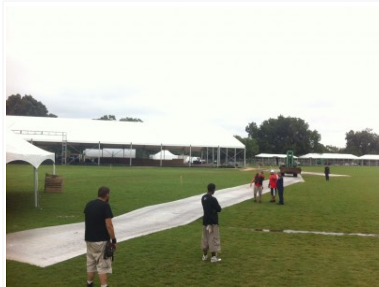
Aluminum "LD" rolls being laid out on festival grounds
