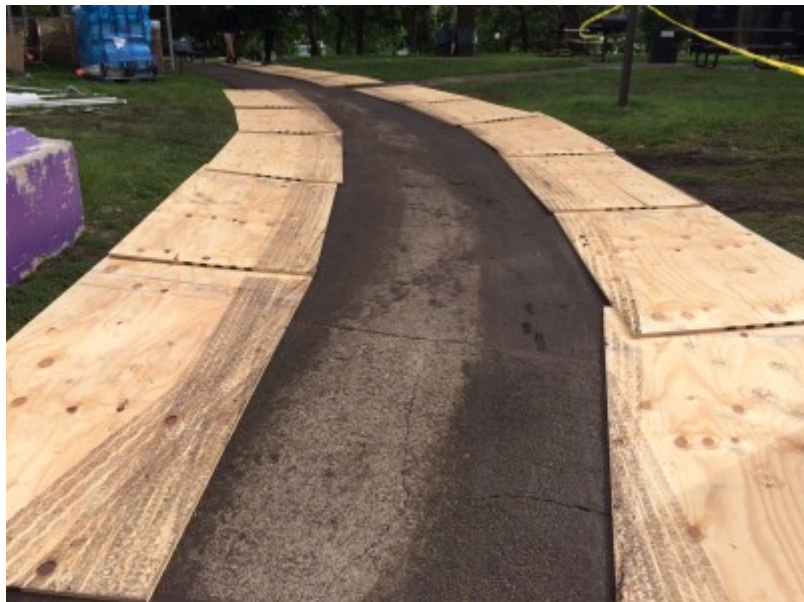
Plywood flanks a backstage access road after a rainstorm
