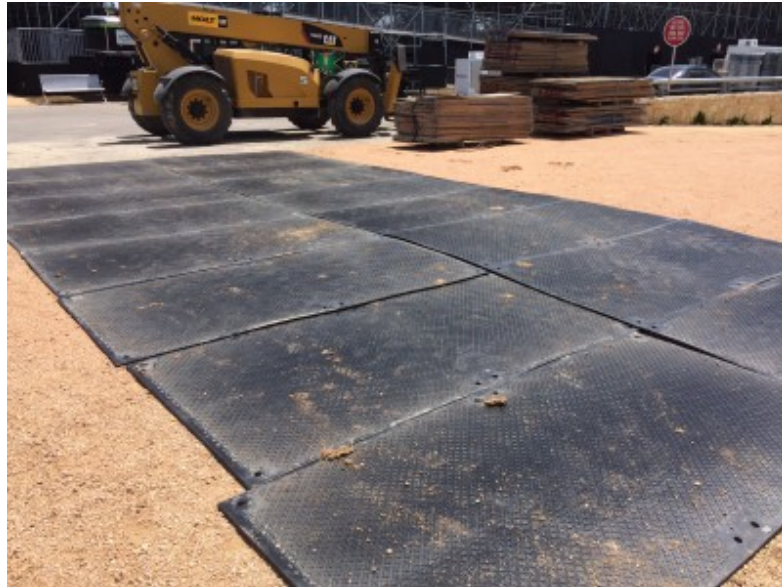
Reusable plastic 4 x 8 ground protection mats
