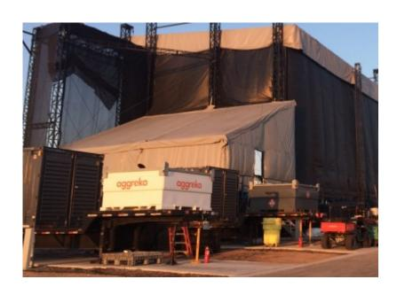
Twin pack 1.5 MW Generators capable of providing electricity to 330 households
