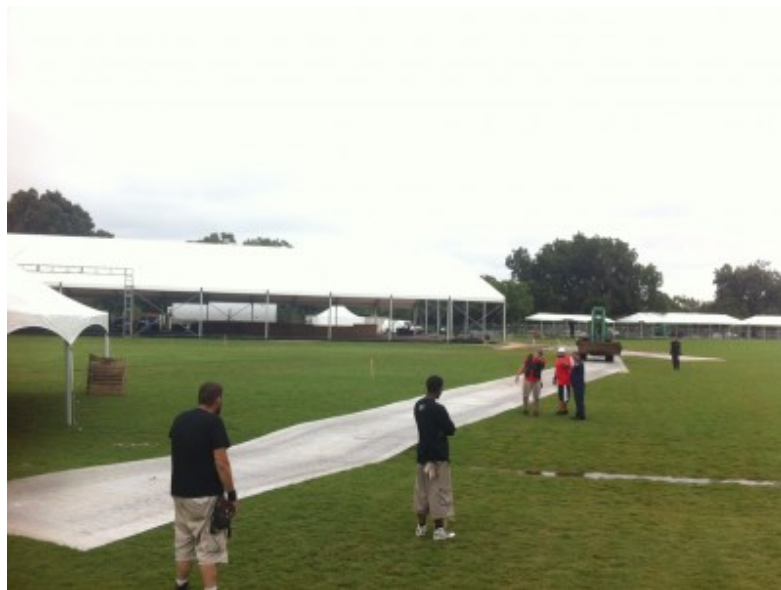
Aluminum "LD" rolls being laid out on festival grounds
