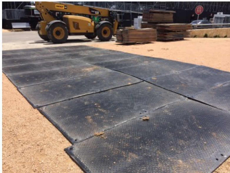
Reusable plastic 4 x 8 ground protection mats
